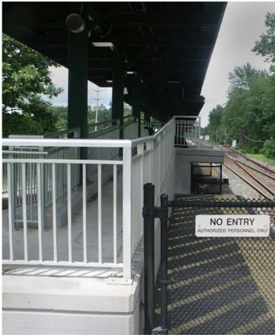
Mini-High Platform with Appropriate Barrier
